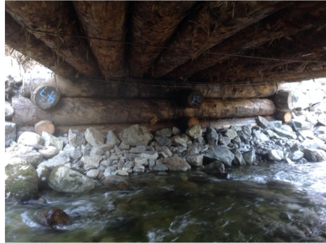
Left Bank Abutment when facing downstream
