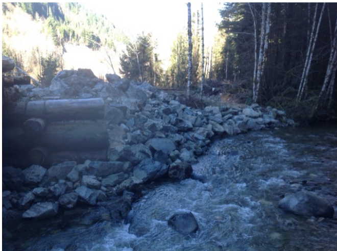
upstream right riprap
