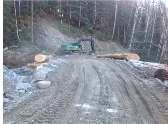
Approach from Right Bank when facing downstream
