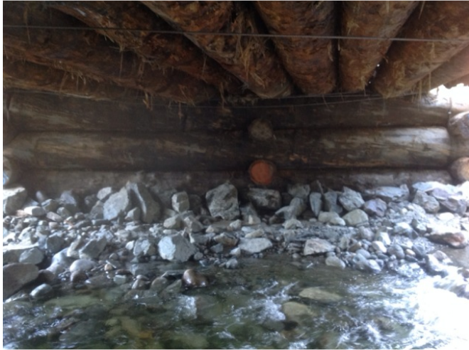
Right Bank Abutment when facing downstream
